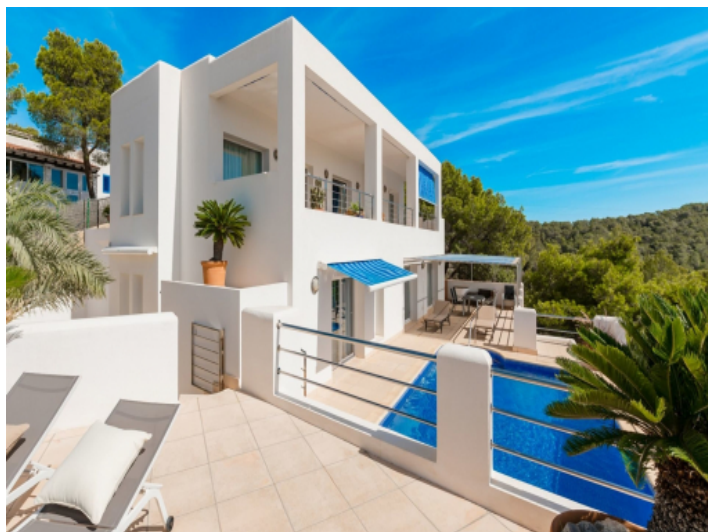
Back façade and pool
