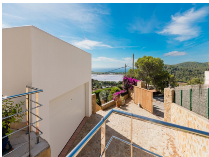
Entrance area and parking space
