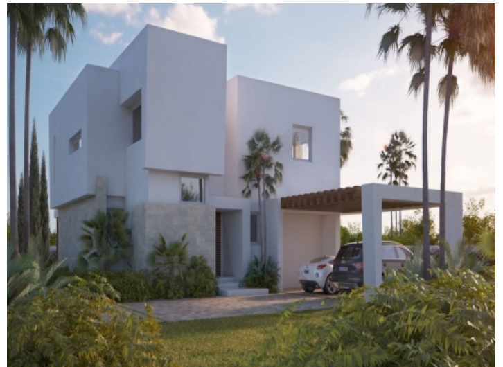
Inviting entrance area with carport
