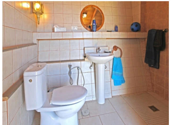
Shower room of the main apartment
