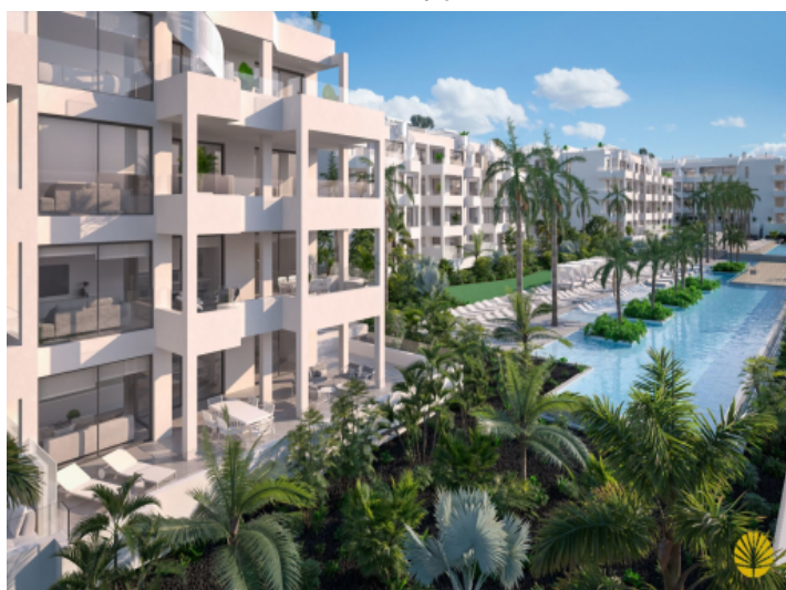
View to the complex
