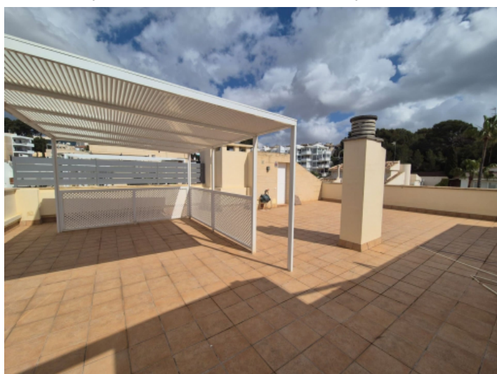
Rooftop terrace with pergola
