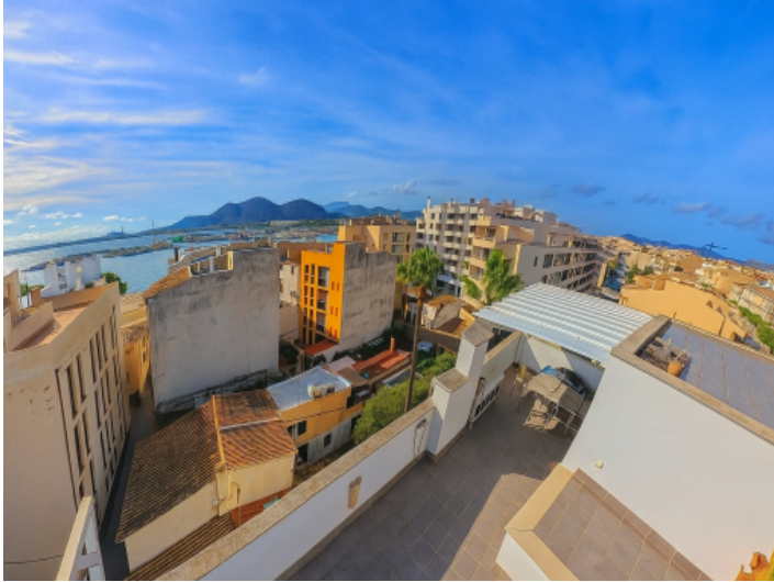
Roof top terrace
