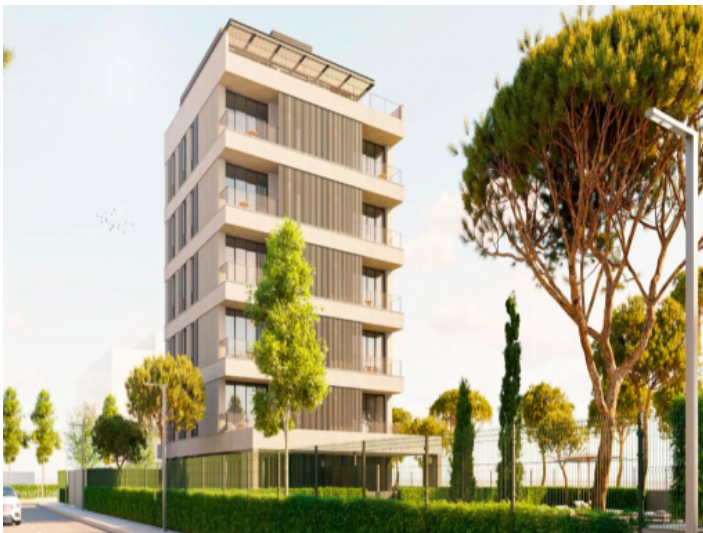
View to the building
