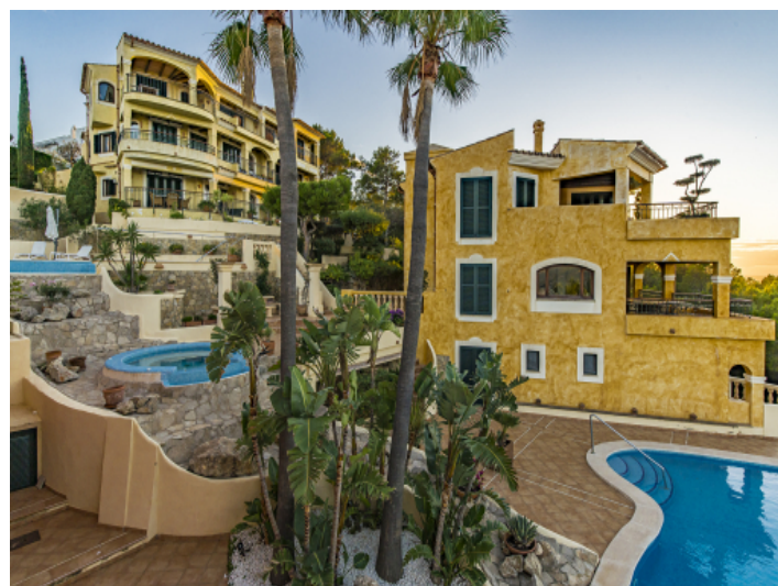
Complex and outdoor area
