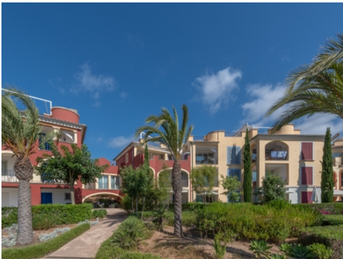
Exterior view of the residential complex
