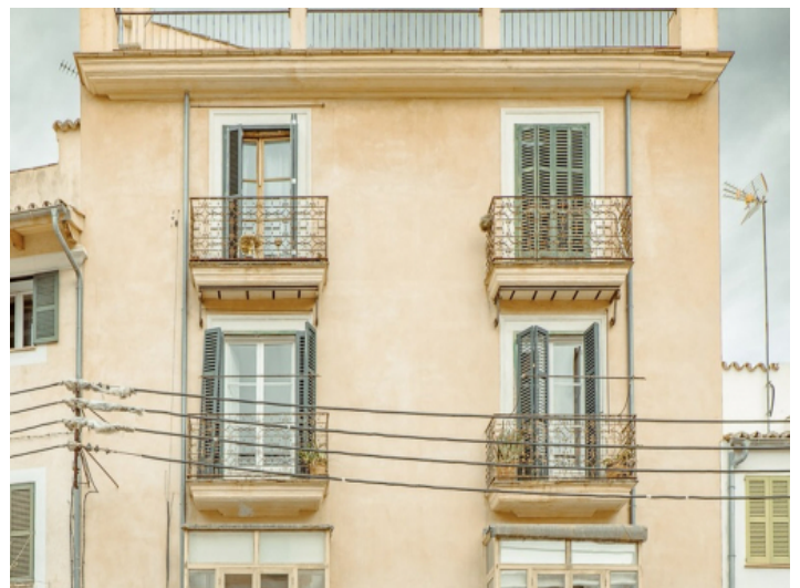
View to the building
