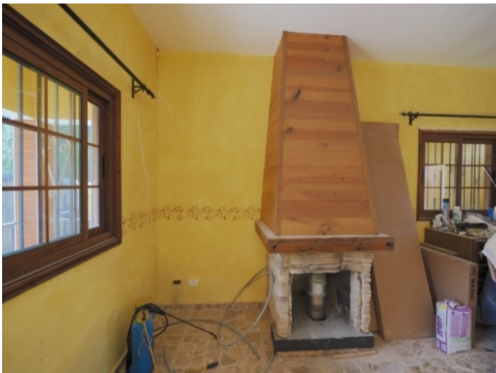
Chimney in living area of main house
