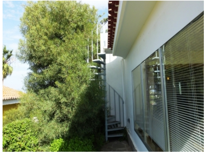
Stairway to the roof terrace
